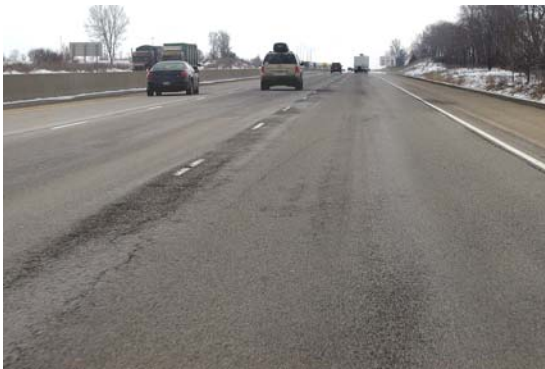
FIGURE 20 Second Generation HIR Section, 2005. Fair to Good Ride Quality With Considerable Ravelling.
