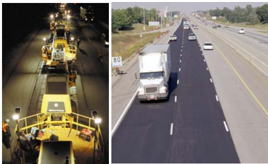
FIGURE 10 Canada – 1999, Ontario Highway 401 Demonstration Project, 5.6 lane-km HIR Section as Part of Five Rehabilitation Strategies Comparison.
