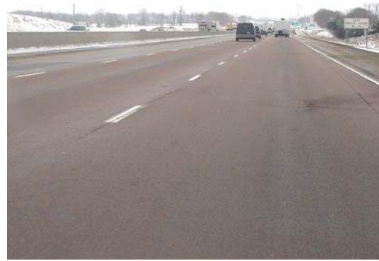
FIGURE 21 Mill and Fill With DFC Section, 2005. Good Ride Quality With Occasional Ravelling and Potholing.
