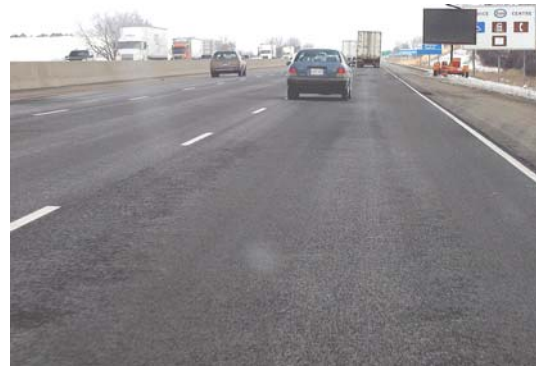
FIGURE 23 Microsurfaced Section, 2005. Good Ride Quality With Very Coarse and Open Texture.
