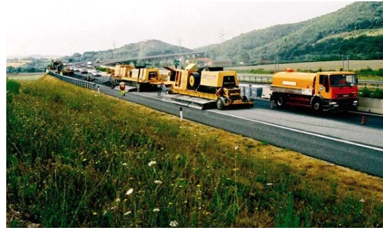
FIGURE 11 Italy – 2003, Livorno – Cecina Section of A12/E80, Combination of Martec AR2000 and Marini ART220 Recycling, Polymer Modified Porous Asphalt (9).
