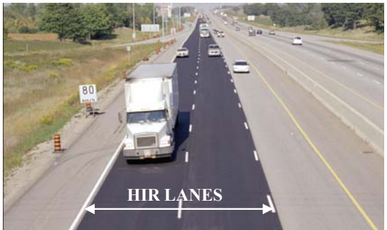
FIGURE 16 Completed Martec AR2000 HIR Section in September 1999 with Typical Highway 401 Truck Traffic on this US-Canada NAFTA Route.
