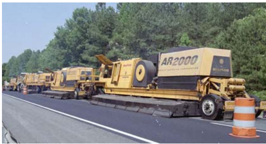
FIGURE 5 Third Generation HIR. Martec AR2000 Full Remix Option, Interstate 85, North Carolina, Open Friction Course, 2001.
