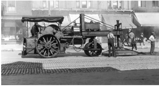
FIGURE 1 Steam Asphalt Pavement Heater Working at Queen and Duncan Streets, Toronto, 1916. (City of Toronto Archives)
