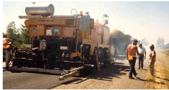
FIGURE 4 Second Generation HIR. Remix Process (No Rejuvenation), B.C. Highway 1 Near Langley, late 1988 (7).
