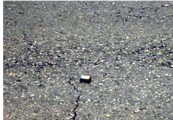
FIGURE 26 Typical Top-Down Cracking (TDC) in Wheelpath, With Some Transverse Thermal Cracking, of Relatively New Expressway Near Hohhot, Inner Mongolia, China.
