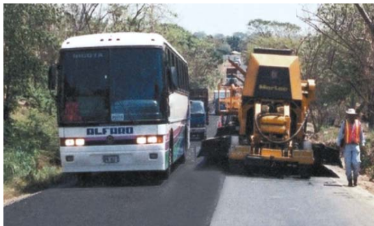
FIGURE 12 Costa Rica – 2004 North Section of PanAmerica Highway, 185 lane-km, to AASHTO 19 mm Surface Course Requirements.
