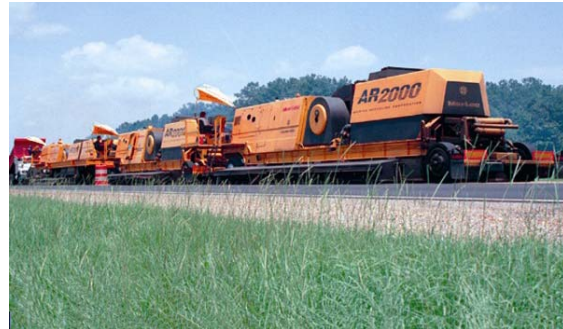
FIGURE 9 United States – 1998, Mississippi Interstate 55, 49.5 lane-km 180,600 m 2 , Re-recycling of Previous Second Generation HIR to Superpave Requirements (10).
