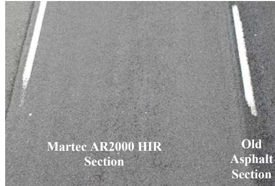
FIGURE 19 Closeup of Martec AR2000 HIR Section. Uniform Surface Texture With No Apparent Deterioration.
